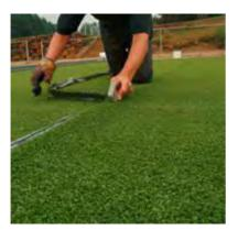
When the grass has been correctly positioned, the seams are cut straight with the long knife. When the whole field has been aligned correctly and all seams cut, the gluing process can begin.
