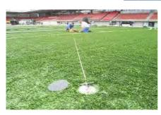
very exactly. Measure the radius from the centre of the circle. Once the turf is 100% complete, check all seams and inlays, and seal with adhesive where necessary.
