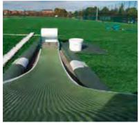
Once the seam is ready for gluing, fill the adhesive box with the adhesive. One person will stay with the adhesive box and guide, while the second person pulls the seaming tape through the adhesive in the box in the seam opening. (When using a two-component glue, one person will work on mixing the adhesive during the gluing process.)
