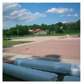
When the grass arrives at the site, it is most efficient to place the rolls directly beside the field. Depending on the equipment available and specific situation, the rolls can be placed along the field with machinery such as a shovel or forklift or manually using a carpet trolley. Take the following into account when placing the rolls along the field:
