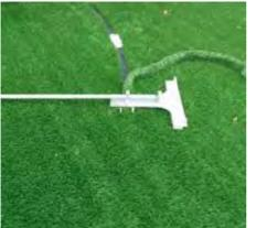
After cutting, the same gluing method is used as with the seams. The only difference is that for inlay lines, a wider adhesive box is used. This is to ensure that the inlay and grass are sufficient affixed to the adhesive. After the goal and penalty area, the sidelines, centre circle and penalty areas can be done.
